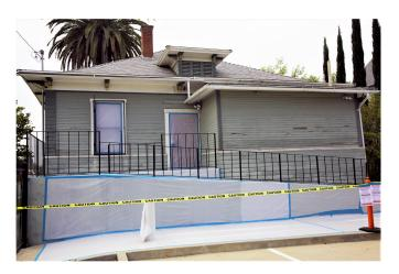
In this photo, the area is beginning to be prepped, with the door and windows taped over and the concrete ramp draped as well. You can see where the existing paint is peeling – it's like that all around the building.
