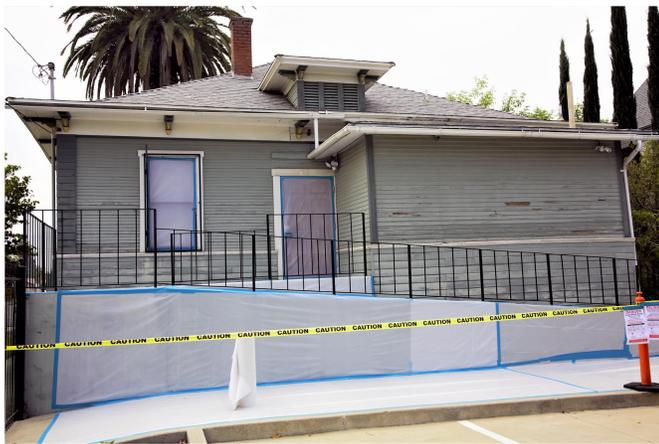
In this photo, the area is beginning to be prepped, with the door and windows taped over and the concrete ramp draped as well. You can see where the existing paint is peeling – it's like that all around the building.
